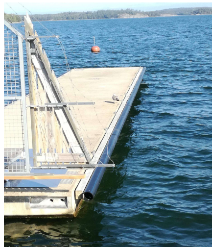
Fig. 5.3 f – Shielding system on a peer. As it is possible see from the picture a hose has been added to a previous but not functional system.
