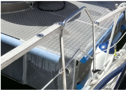
Fig. 5.3 e – Two floating stations: The station on the left has no shielding system on the edge which can cause aesthetic or more severe damages to the boat.
