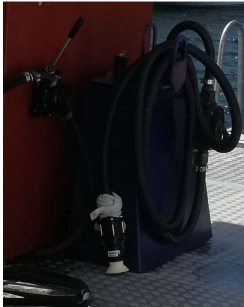
Fig. 5.3 c – The hose nozzle of this floating station is equipped with a sucker, that makes it easier to have a vacuum condition.
