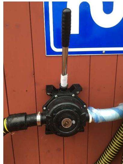
Fig. 5.4 – Floating pump-out station in Finland: The steps on one side allow easy access to boats with different heights. This pump-out station is equipped with a hand-pump and the tank is inside the pontoon.
