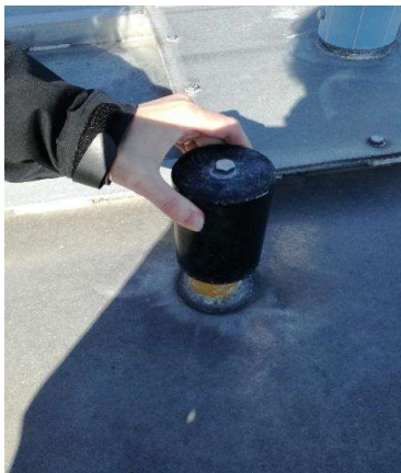
Fig. 4.4 d - Örö floating pump-out station. In the third picture it is possible to see the mechanism that indicates when the tank is full.
