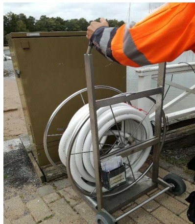
Fig. 4.4 c - Sewage collecting system in Nauvo. In clockwise order: the pier, the suction point, the portable hose, the pump station.
