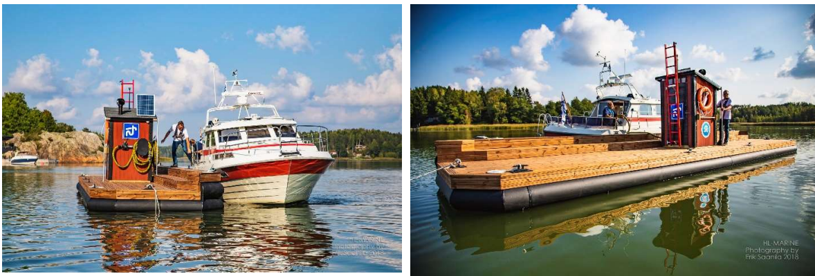
Fig. 5.3 d – Floating pump-out station in Finland: The pontoon has steps on one side in order to make it easily accessible to higher boats.
