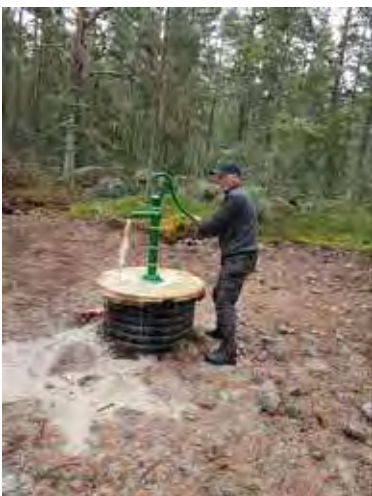
Picture 56. The fresh water well is 6m deep in total and the water level is 50-100 cm. © Per-Olov Persson
