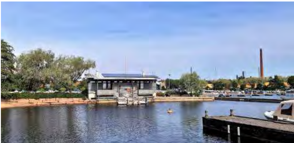
Picture 20. Sapokka's new solar power plant in August 2021. © Jussi Sutela
