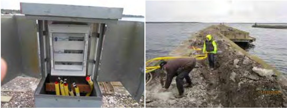
Pictures 35 and 36. The Sub-fuse box on quay and cable installations. © Leif Ortman
