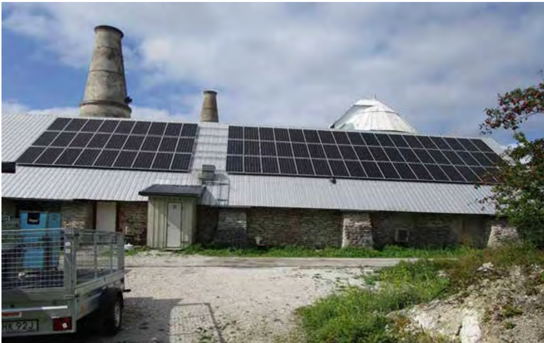
Picture 34. Bläse Kalkbruk restaurant building with 31.6 kWp of panels installed. © Leif Ortman
