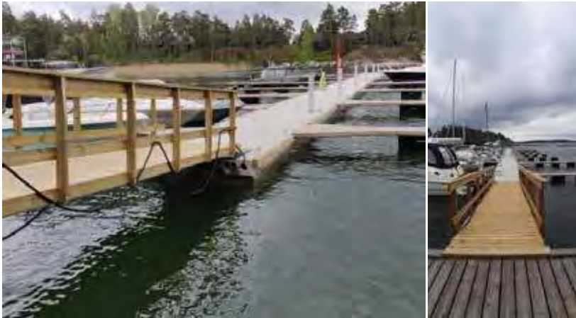
Pictures 10 and 11. Two new concrete pontoon guest piers in Airisto Marina. © Teemu Heikkinen
