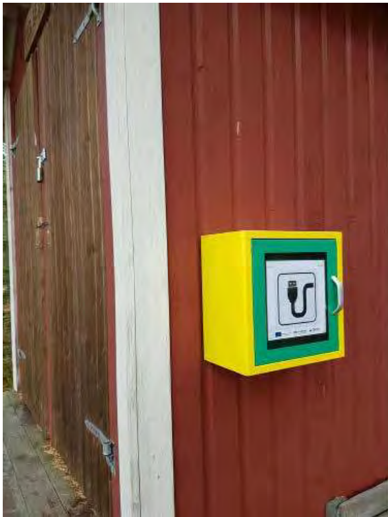
Picture 52. Northern pier: Box with sheltered USB-socket for charging mobile devices. © Per-Olov Persson
