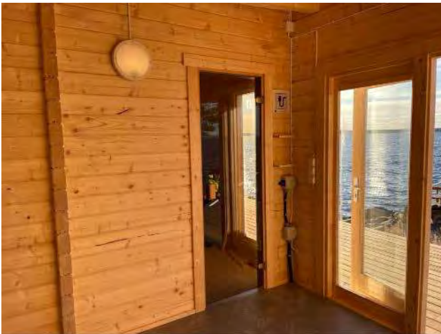
Picture 55. Southern pier: The newly built sauna was equipped with lighting and USB-socket. © Stefan Lindgren
