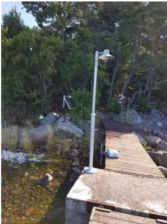
Picture 53. Northern pier: Solar cell on a special mounting and safety lighting at the gangway. (Toilet building in the background) © Per-Olov Persson
