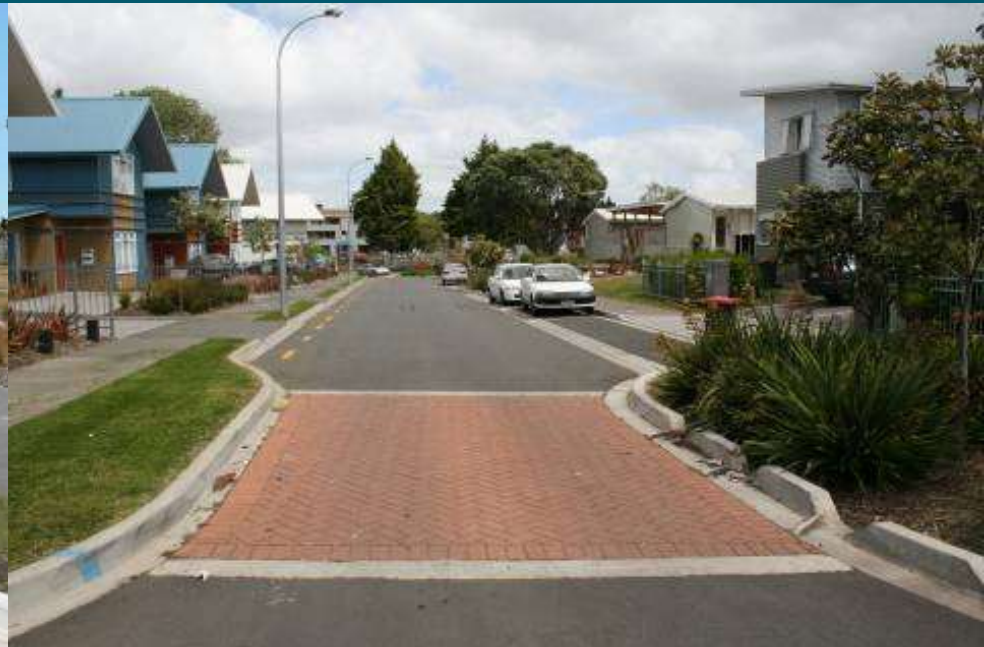
Narrow Road, Talbot Park subdivision, Auckland. Rain garden on right treating road runoff and forming a traffic-calming feature
