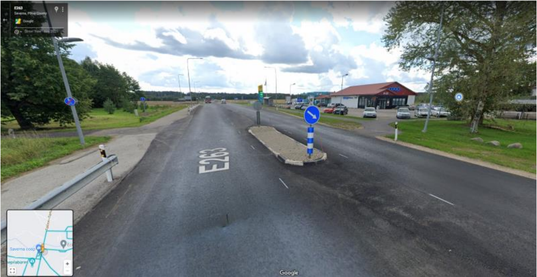
Figure 4 Safety island on E263 near Saverna
