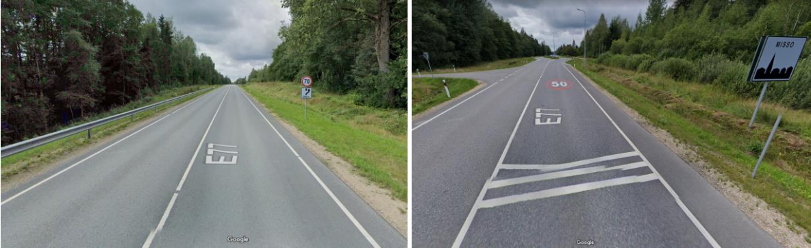
Figure 13 Speed reduction measures on E77 before village and before chicane
