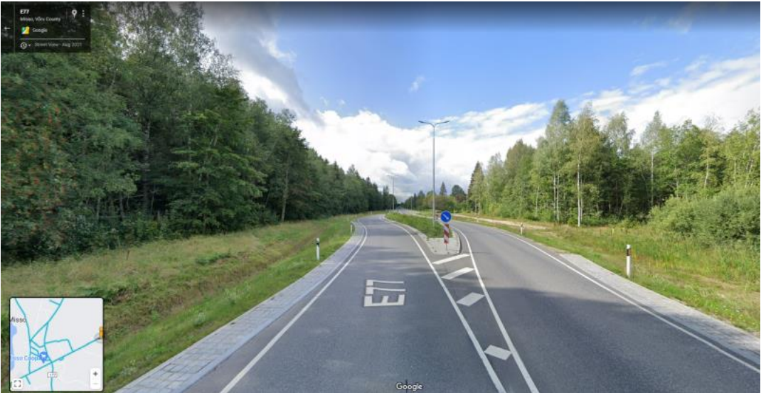
Figure 5 Safety island and chicane on E77 near Misso
