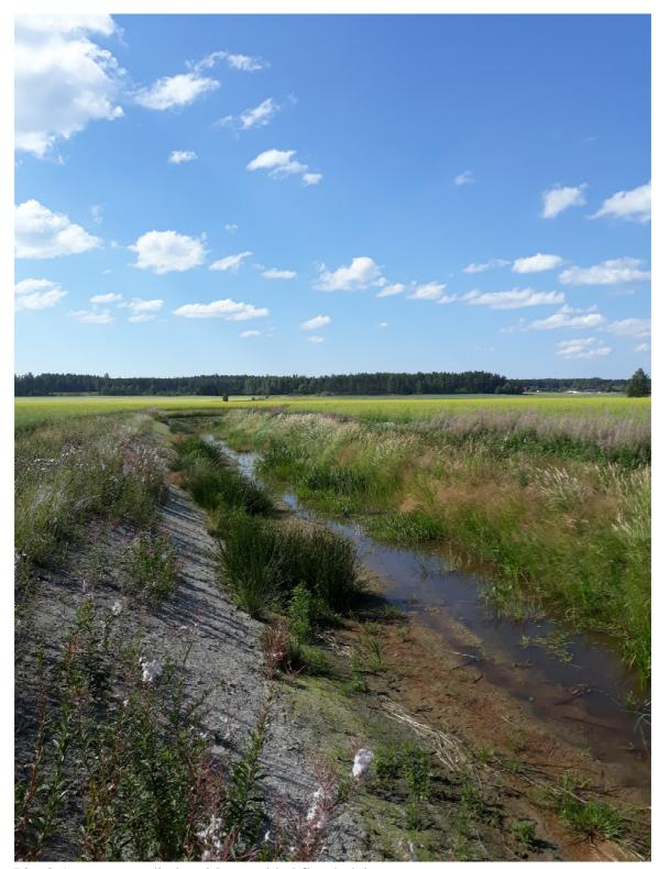
Pic. 2 A two-stage ditch, with one sided flood plain
