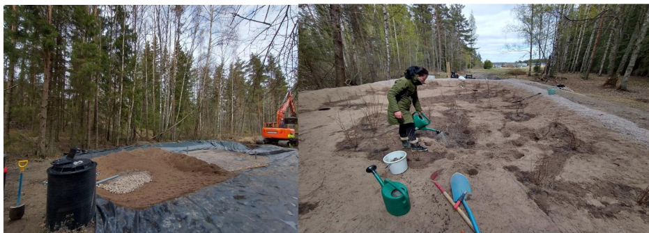
Installation of the filter medium (left) and watering of newly planted vegetation at the Lieto pilot (right).
