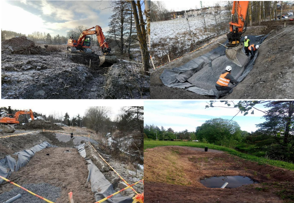
Construction of the Turku pilot site in December 2021 (top) and the ready bioretention basin in May 2022 (bottom right).
