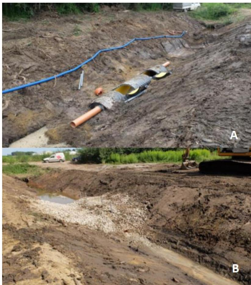
Figure 1. The small-scale P filter. A) The filter with inlet/outlet pipes; B) The functioning filter with the sedimentation basin.
