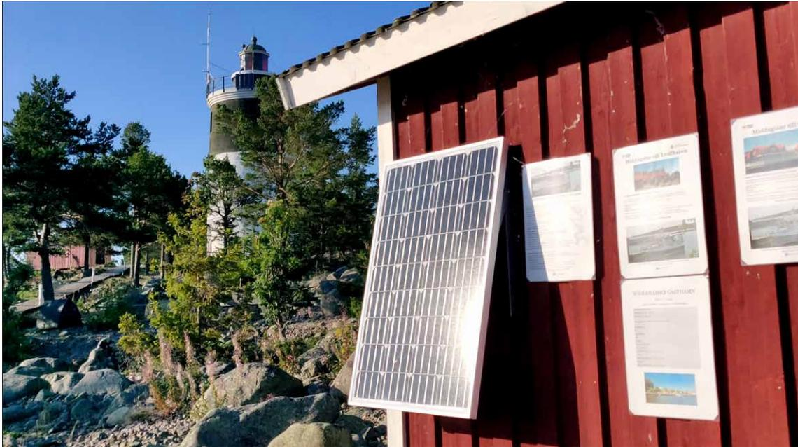
Figure 20. Fyrhamn port in Storjungfru island in Söderhamn is not connected to the grid. An off-grid PV system was installed as an PortMate investment. © Alberto Lanzanova
